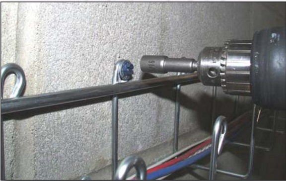
Figure 6 - Wall Snake attached directly to the wall using CM-501-CA anchor bolts
