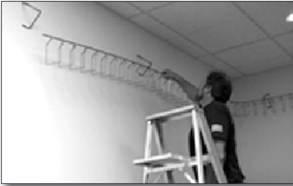
Figure 4 - Installing Snake Tray on a wall using WBN wall brackets.
