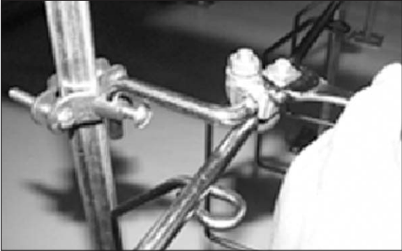
Figure 5 - Securing the 201 Series Snake Tray under an access floor to the vertical pedestal base using the ST-201 bracket.
